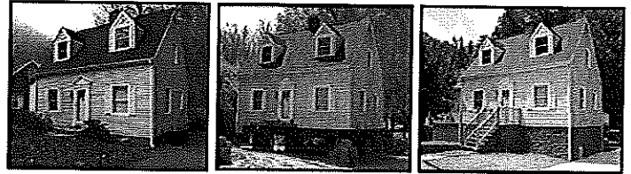
An elevated structure with flood vents
